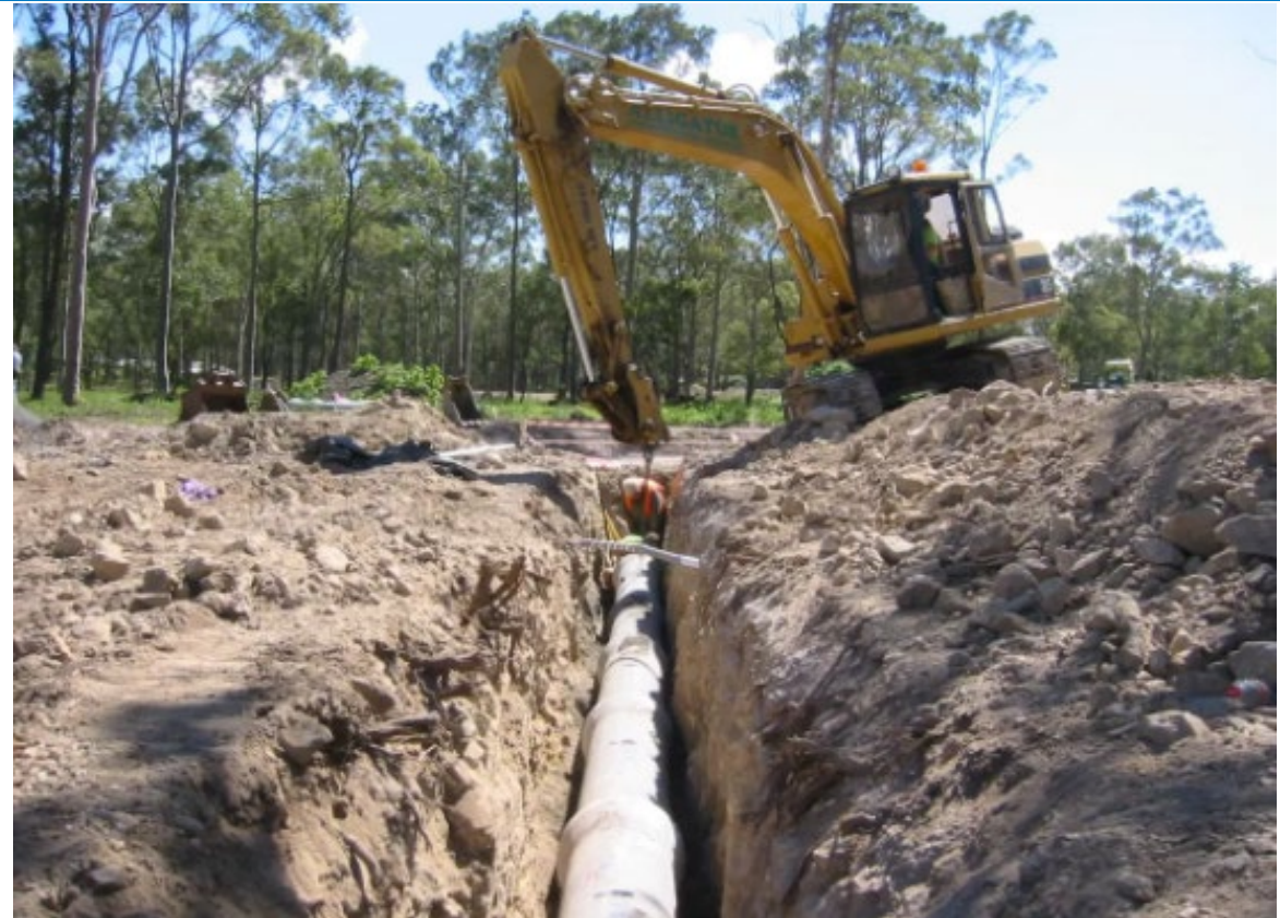
Open Cut installation ~5m wide clear cut area
