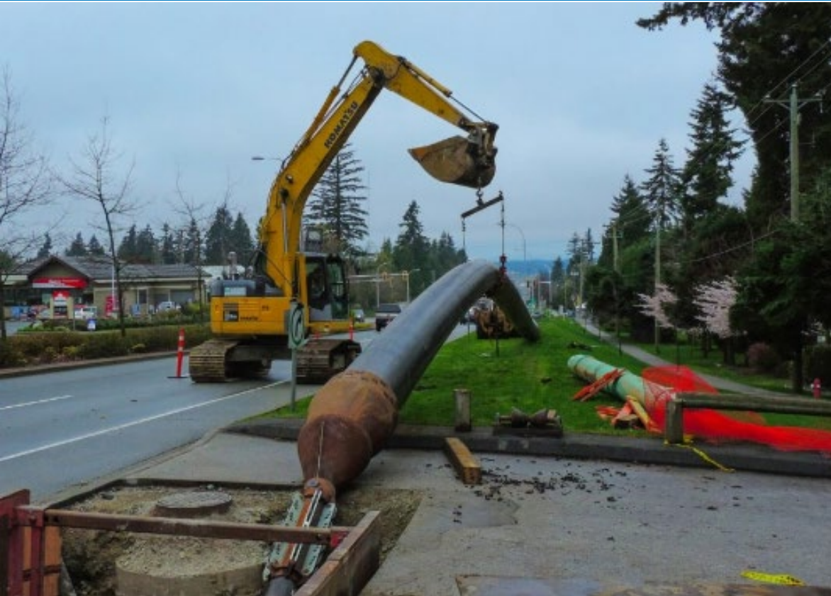
Trenchless installation 15 - 6x3m pits
