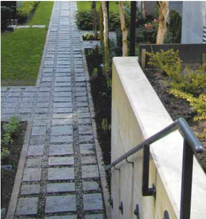
Unit pavers allow infiltration of rain water
