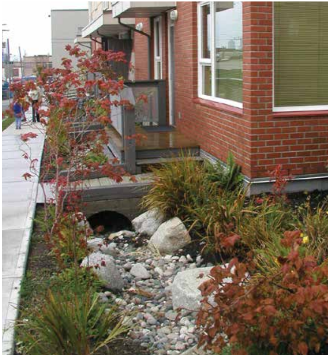
Image showing the use of pervious materials and Naturescape planting in support of stormwater infiltration and habitat enhancement.
