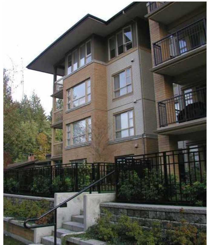
Example of West Coast architectural expression. Key elements include: generous roof overhangs, low sloping roofs, generous glazing, the layering of materials, simple detailing, an emphasis on horizontal lines and the use of warm, natural colors.
