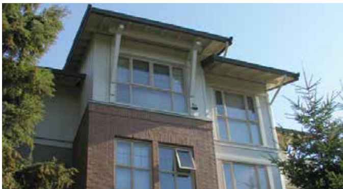
Examples of buildings with generous roof overhangs that provide shade and horizontal emphasis.
