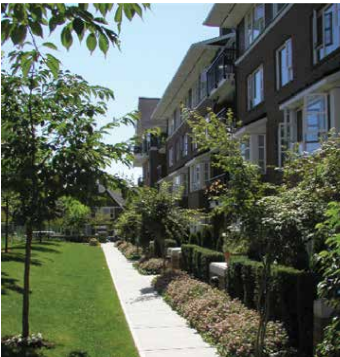
Example of a common greenway separated from private backyard space with low walls and planting.
