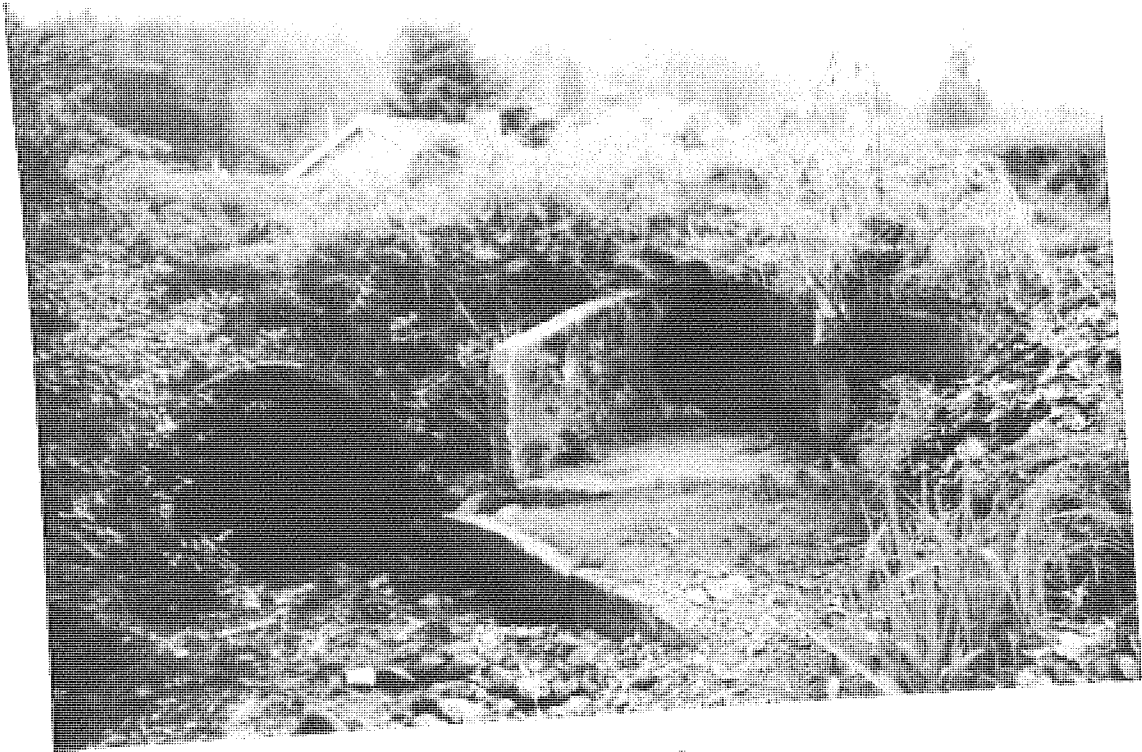
Reach S12 Inlet structures at Clarke Street crossing 1500 dia. woodstave pipe. 900 dia. concrete overflow.
