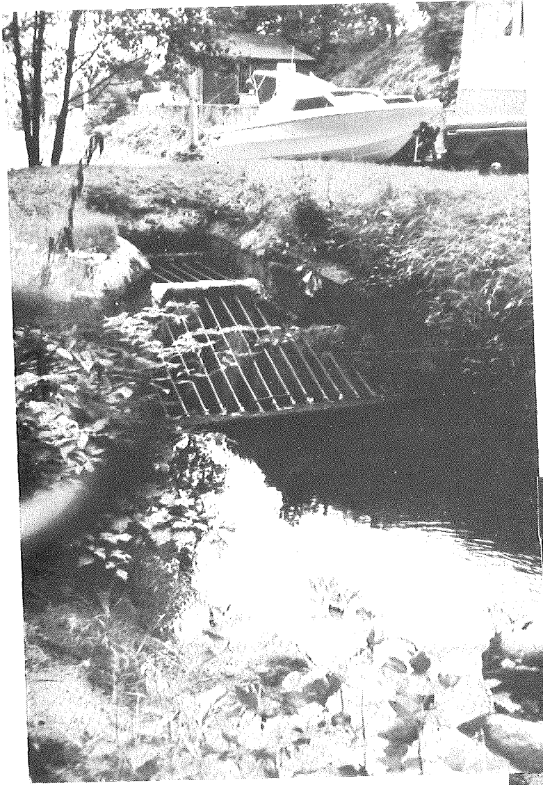
Sundial Creek channel, sediment traps, trash guard pickets and intake in Kyle Creek Drainage Area.
