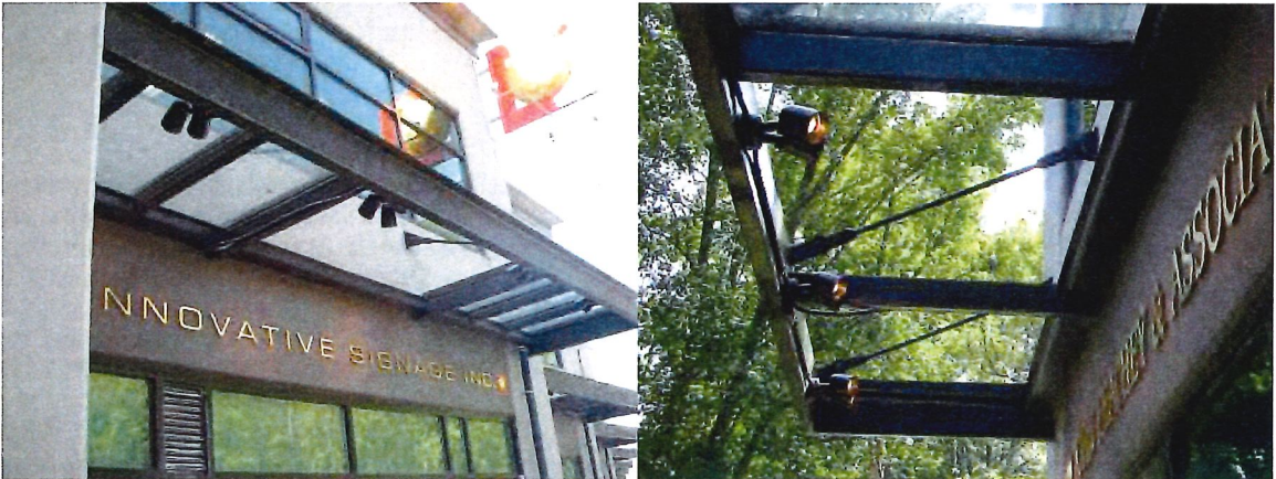
Lighting from under canopy for non-illuminated fascia signs
