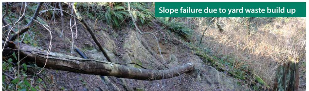
Slope failure due to yard waste build up
